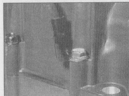
26.12b ... one bolt secures a ground wire ...
